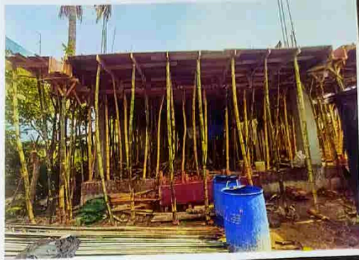
Under construction House
